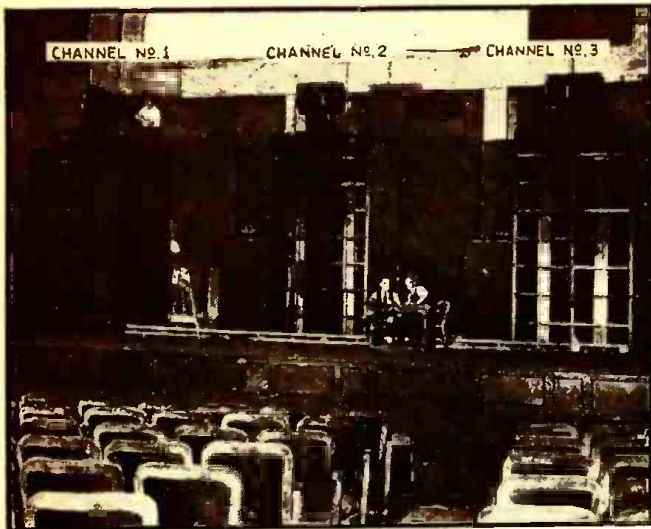
The 3 special super-power high-fidelity loudspeaker assemblies in back of the picture screen on the theatre stage. A heavy hair-cloth curtain in back of the speakers absorbs the back waves. Each 15-ft.-high bay includes a group of 8 L.F. speakers topped by a 4-horn-unit honeycomb-type H.F. projector. (See Fig. 1.)
